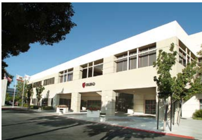
Gilead-Gebäude (Headquarter in Foster City)
